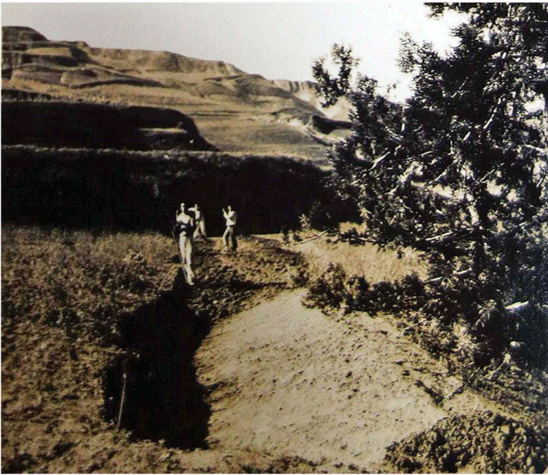
Figure 3. Digging broad-based ditches.
